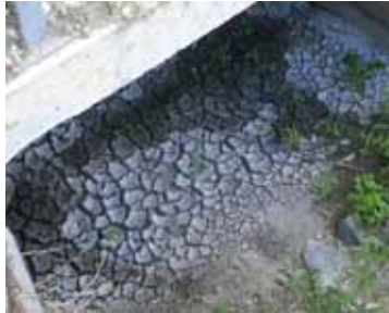
Figure 5-12 a) to c): Examples of clogging processes detected in the rafts and channels "artificial recharge" predominant physical processes
