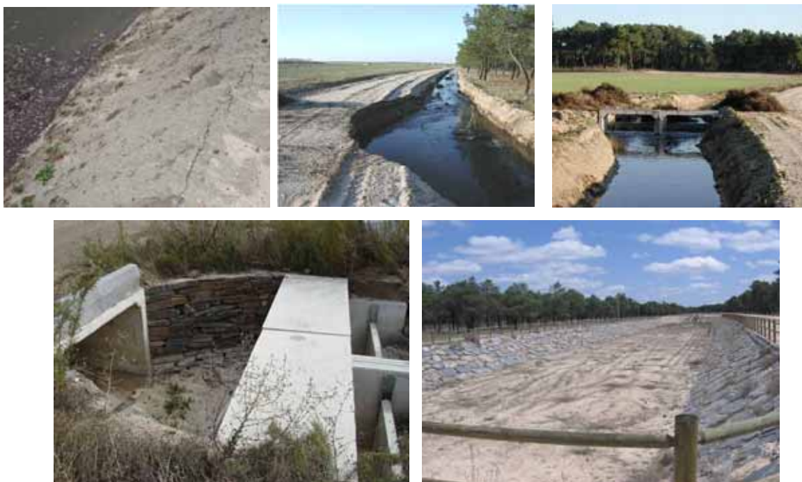
Figure 6-10 a) to e): 1:1 slope with potential slices due to desiccation processes (a, b); 2H:3V initial design (c); 3H:2V as the most common slope in the channels and ponds walls (d); and eventual gabions protections (e)
