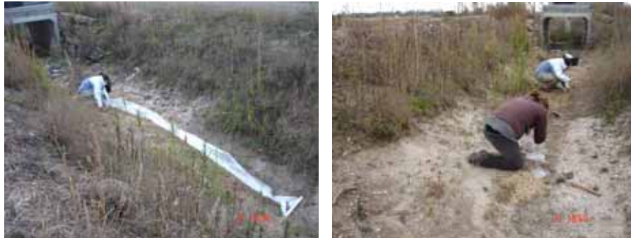
Figure 6-11 a) and b): Geotextile installed in the bottom of the channels to facilitate the cleaning of clogging processes with minor changes in the infiltration rates
