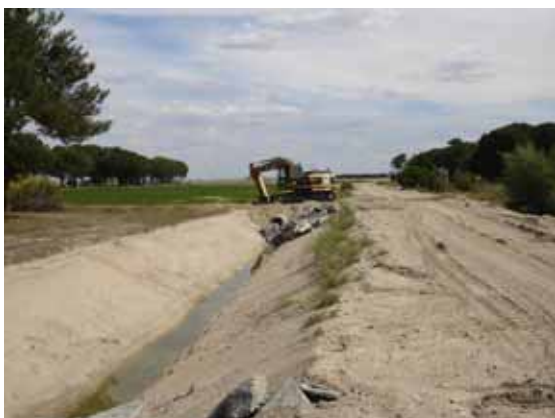
Figure 6-22: Cleaning and maintenance operations in ponds and canal by means of excavators and tractors with adapted accessories
