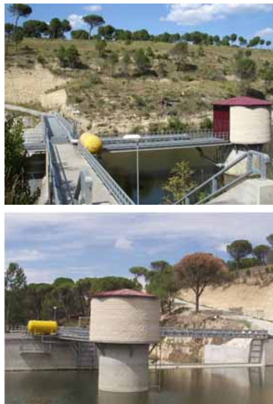
Figure 6-1 a) and b): Ranney well using a River Bank Filtration (RBF) system for water supply from which surpluses are applied for MAR in Santiuste Basin
