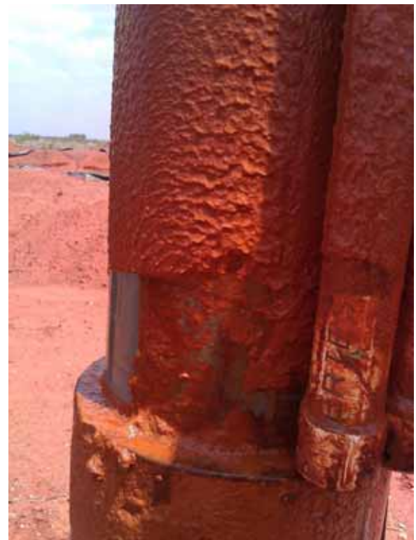
Figure 9: Sediment (introduced from the pipeline system) coating the injection unit
