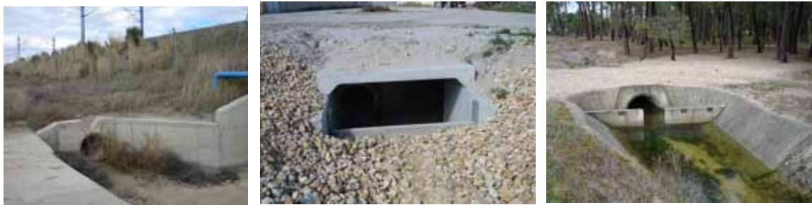
Figure 6-4 a) to c): Run-off traps, stagnation and decantation structures to pre-treat runoff water prior reaching MAR facilities
