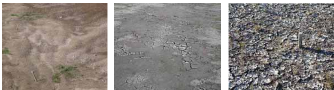
Figure 5-10 a) to c): Clogging deposited in microtopographical depressions at the bottom of the infiltration pond due to self-mulching effect
