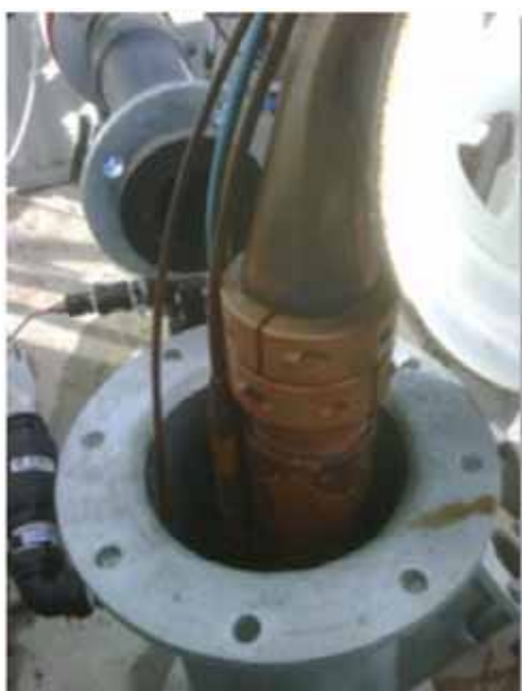
Figure 5: Iron bacteria coating pump collar and rising main. Colonisation occurred within 4 weeks of the pump installation
