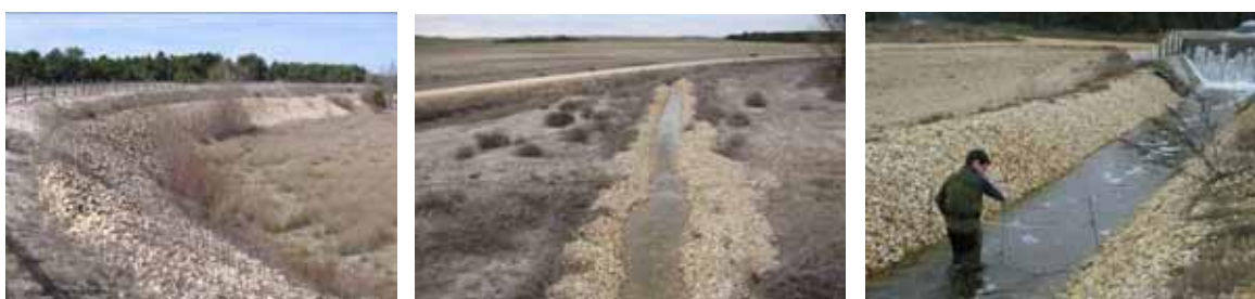
Figure 6-12 a) to c): Gravel filter to result in pH corrections as well as provide stability to some MAR facilities
