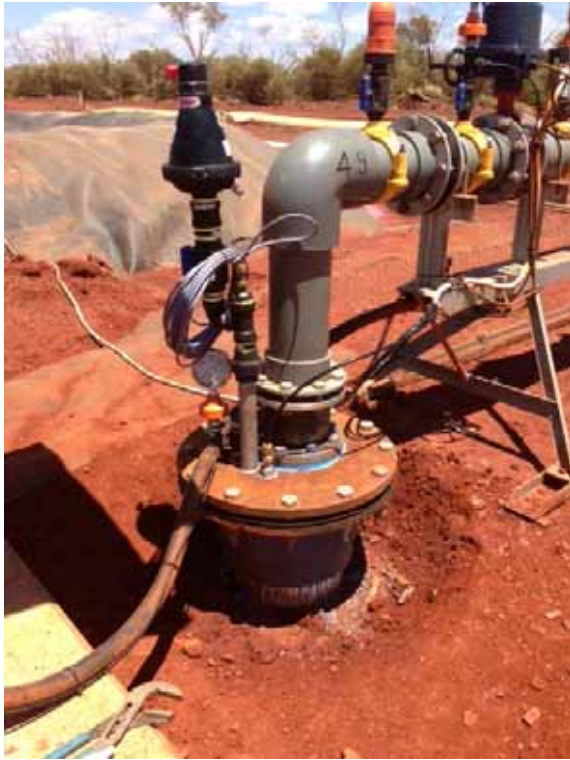
Figure 8: Typical saline injection headworks
