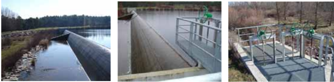
Figure 6-2 a) to c): Dams specially designed for water filtration and pretreatment in one side's specific facilities (filters and a decantation system). Santiuste Basin catchment dam (a-c. Some of the designs applied are inspired from the works of Bouwer (1999 and 2002) and Olsthoorn (1982)
