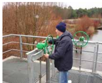
Figure 6-13 a) and b): Manual control of the inlet valve by farmers advised. Close on flood, storms, frost, etc.
