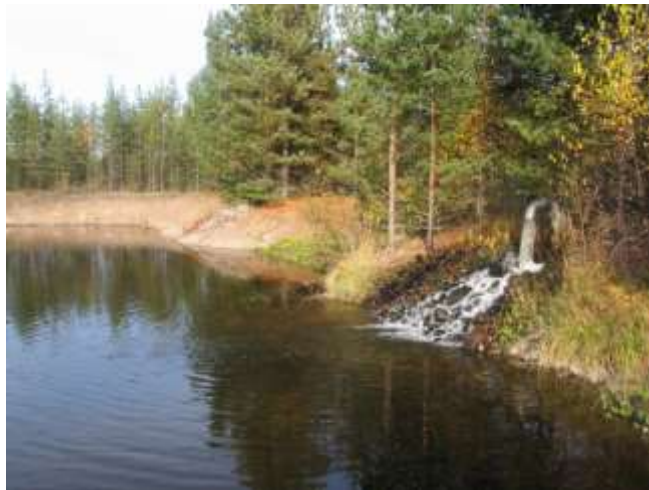
Figure 2. Basin infiltration in summer. On the right: inlet with cascade aeration.
