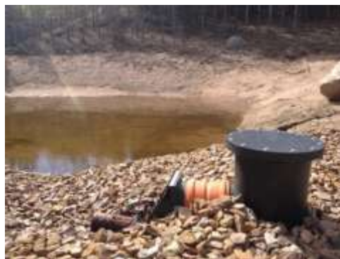
Figure 6. Combined basin & well infiltration at the Jäniksenlinna plant: an infiltration well on the right with an overflow connection to the infiltration basin.
