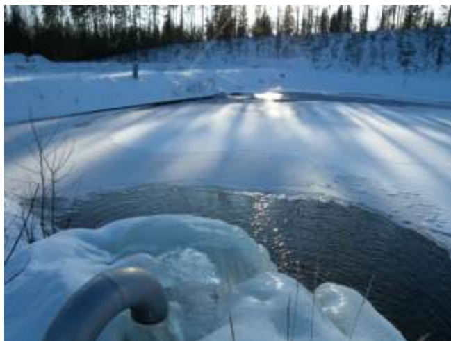
Figure 3. Basin infiltration in winter.
