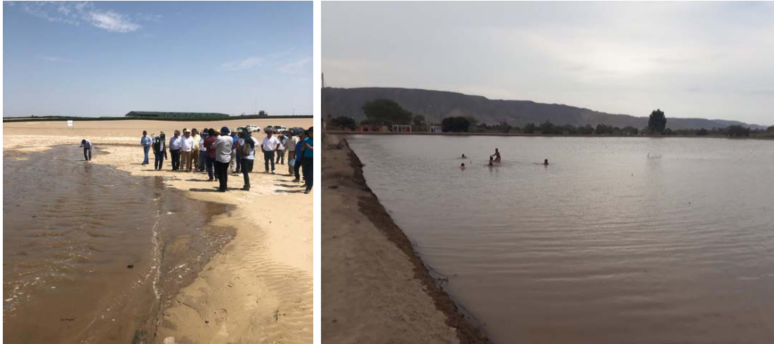
First day of the new infiltrations ponds announced to the press. Photo: Roberto Ramírez Public use (banned) in an infiltration pond. Photo: Roberto Navarro
