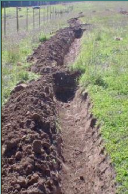
INFILTRATION DITCHES HIDANGO (CHILE.2005)
