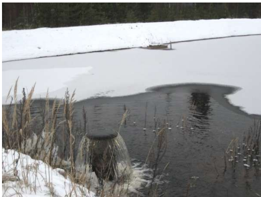
Basin infiltration during winter
